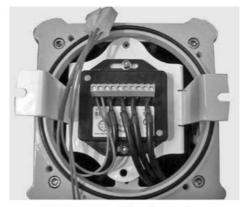
SL10 AMP Regulator shown when correctly fitted
